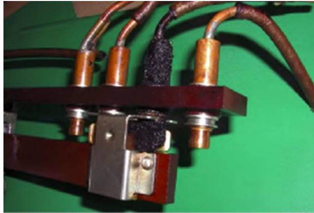
Fig. 6. The result of maintenance on-site [16]
