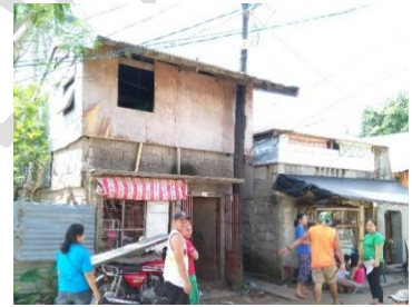
c. Poor building
