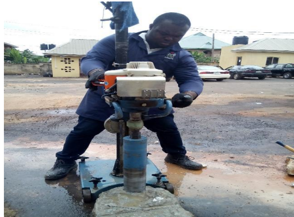
Plate 3: Coring of the concrete mass sample.
