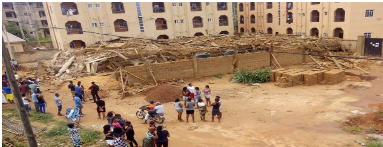
Plate 1: Picture of the 3-Storey- Collapsed Building at Oko, Anambra State Nigeria.
