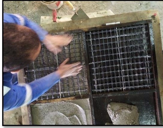
b. shows fixing the reinforcement
