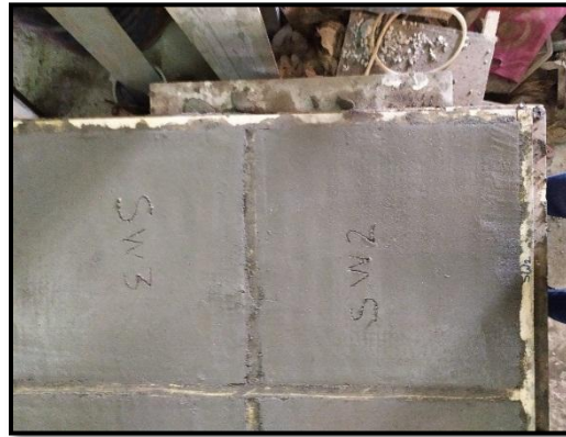
d. shows leveling the mortar surface layer.
