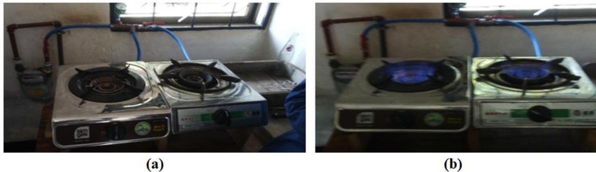
Fig.8. (a) Installed biogas stoves that are turned off when not in use. (b) Installed biogas stoves that are turned on when in use.
