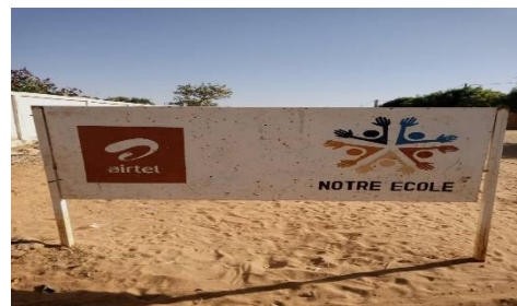
Picture 2. Primary school built by Airtel Niger
