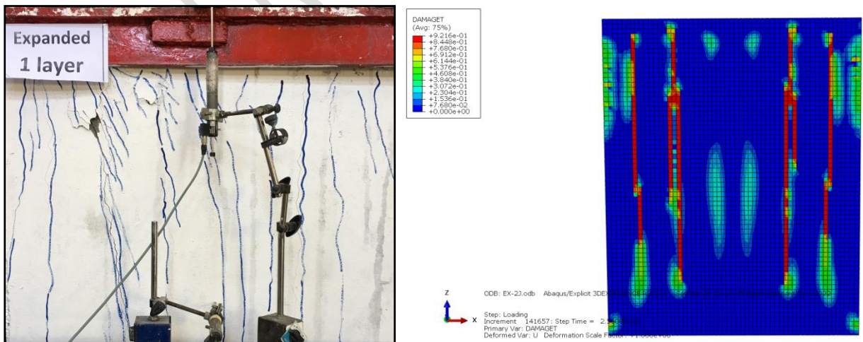
Fig. (32): Experimental and analytical crack patterns (EX1) specimen.
