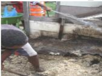
Figure 5. Mixing of the soil and sawdust.
