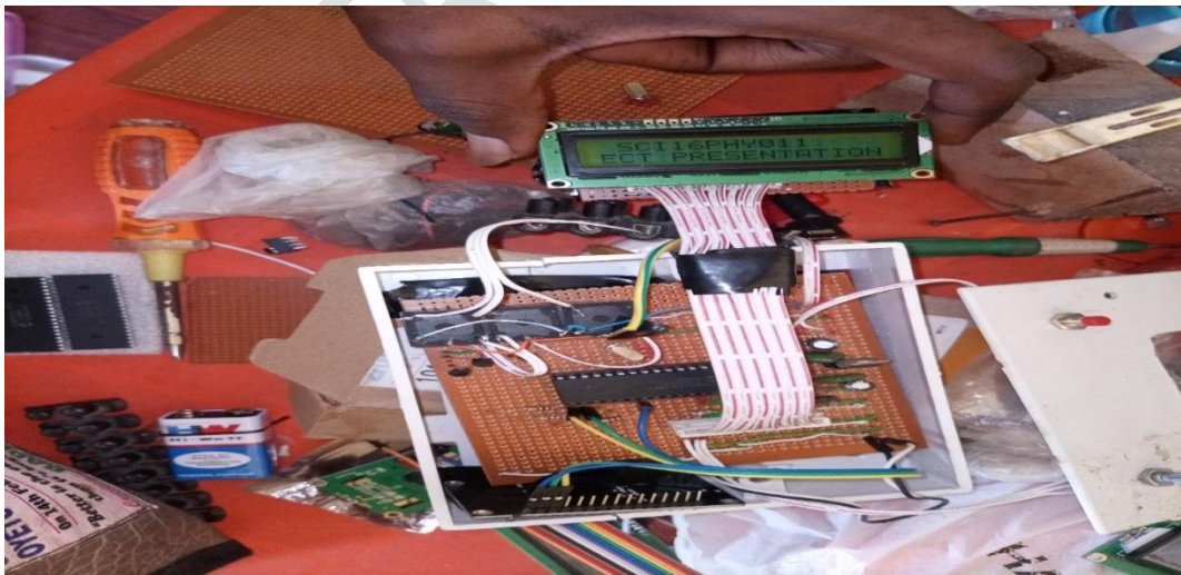
Figure 9: Inside view of the smart-home automation system
