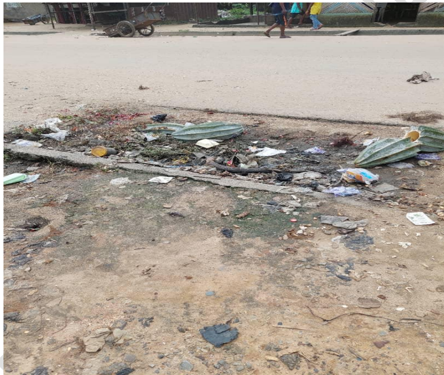
Plate 1: Debris filled drainage in Umuechem Community causing flooding on the adjoining Farmlands Source: Authors' Fieldwork, 2022
