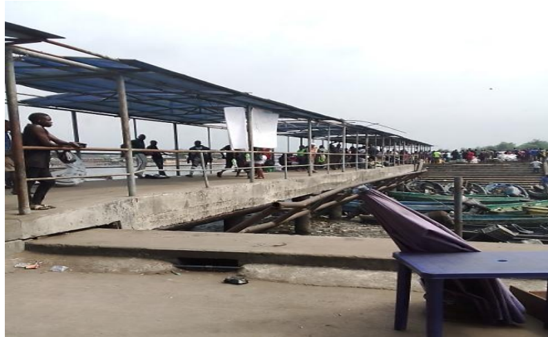
Figure 4: Bille/Bonny/Nembe Jetty, a Newly Improved Water Transport Infrastructure Source: Researcher's Survey, 2021
