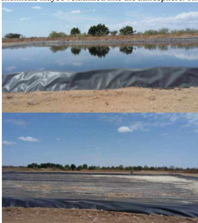
FIGURE 6: EVAPORATION PONDS FILLED WITH SILICATE WATER FIGURE 7: AFTER EVAPORATION OF THE SILICATE WATER
