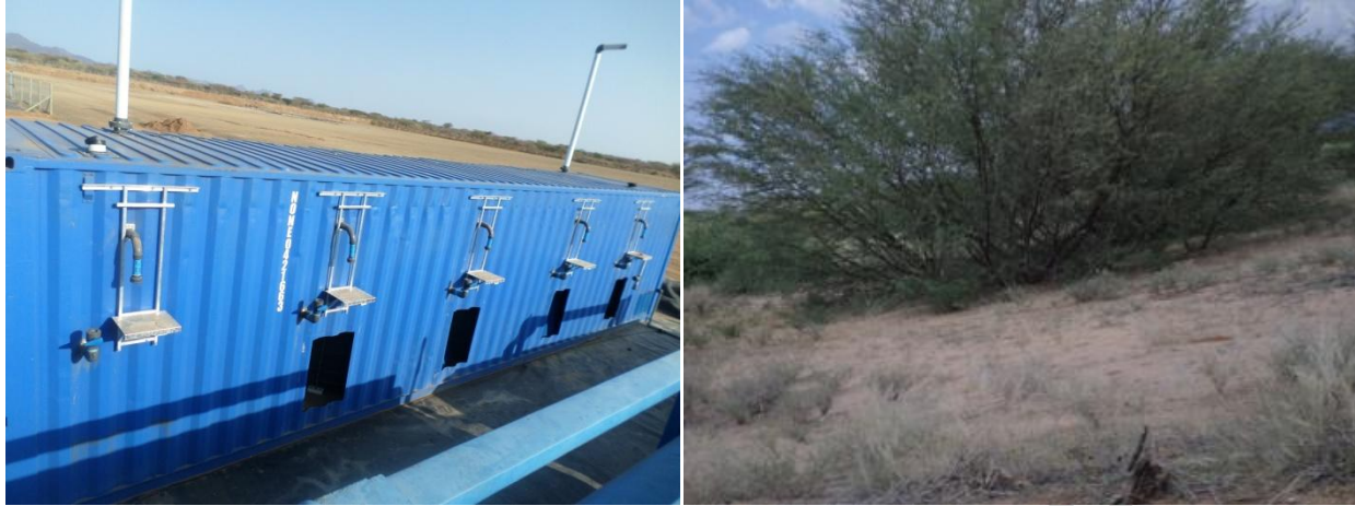
FIGURE 9: EFFLUENT TREATMENT BIO-BOX AND VEGETATION IRRIGATED BY TREATED WASTE WATER
