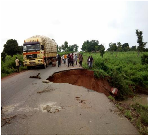
Picture: Jos – Abuja Road
