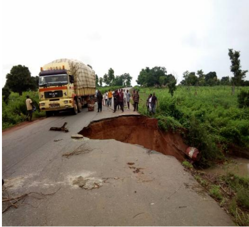
Picture: Jos – Abuja Road
