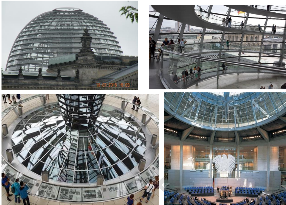
Figure 7. Interior and exterior views of the added transparent dome above the parliamentary hall [URL-4] (Sirel, 2015)
