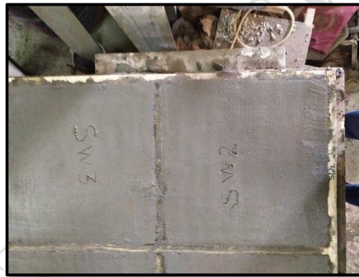
d. shows leveling the mortar surface
