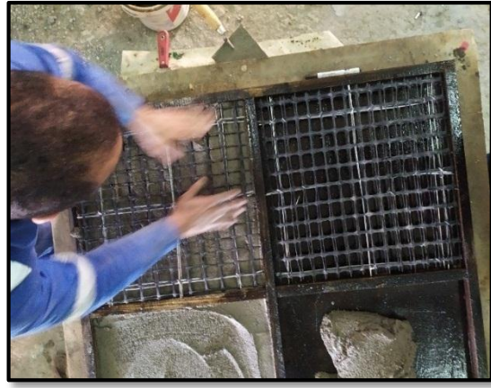
b. shows fixing the reinforcement
