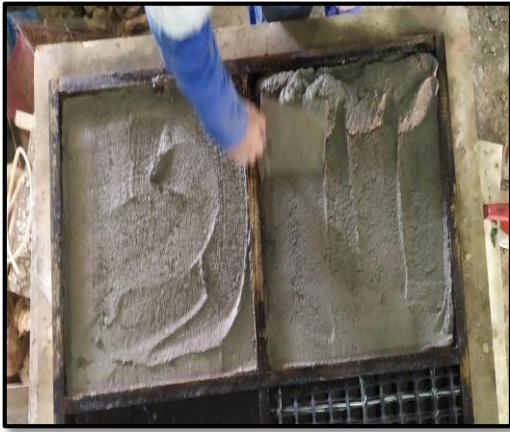
a. shows casting of the bottom skin ferrocement layer
