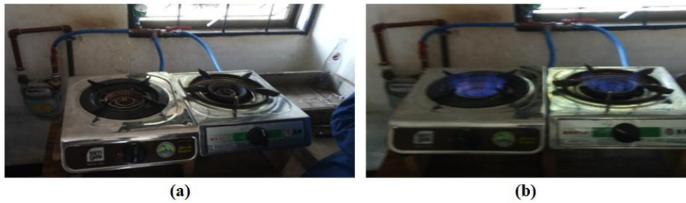
Fig.8. (a) Installed biogas stoves that are turned off when not in use. (b) Installed biogas stoves that are turned on when in use.
