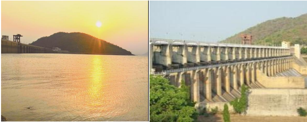
Image 1: (a) Upstream, the Rengali Reservoir and (b): the dam downstream (PH: extreme right, over flow section in the middle and non-overflow in the left flank)
