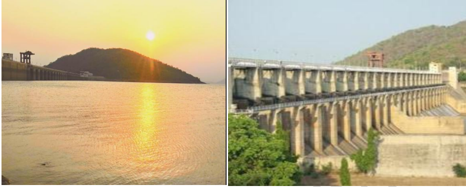
Image 1: (a) Upstream, the Rengali Reservoir and (b): the dam downstream (PH: extreme right, over flow section in the middle and non-overflow in the left flank)
