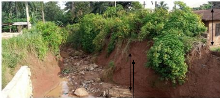
Plate F: The same gully erosion at Onuiyi Road Culvert in 2020 (Note the house around the gully site, with the height of the house about half of the gully depth at 3.84 m)
