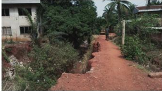
Plate H: Gully cut at Ibeziako Street with the street reduced to a footpath and house endangered by the gully in 2016
