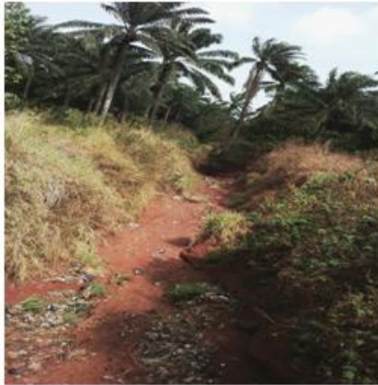
Plate C: Gully erosion section at Onuiyi in 2016
