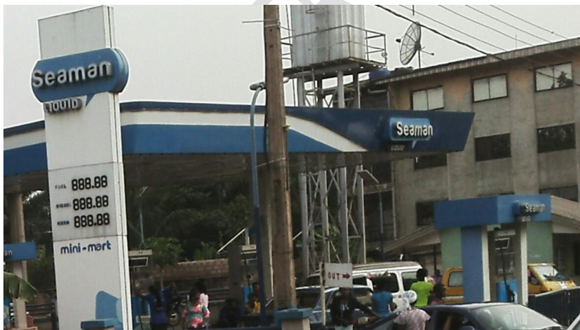
Fig 8: A Filling Station around a high populated residential area
