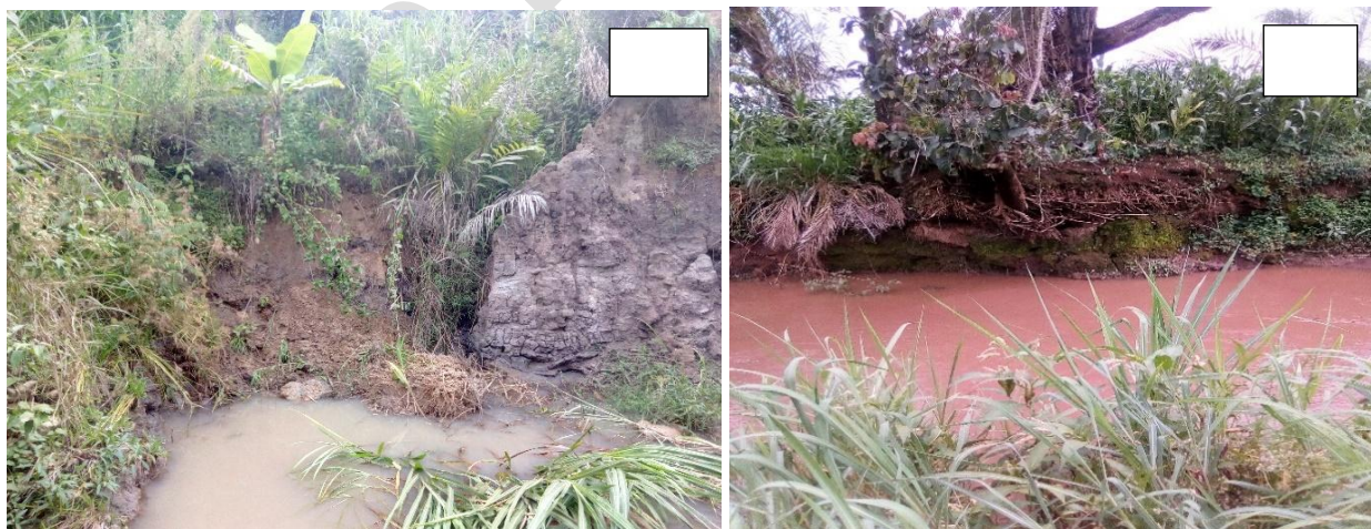
Figure 10: Upper Noun River erosional activities
