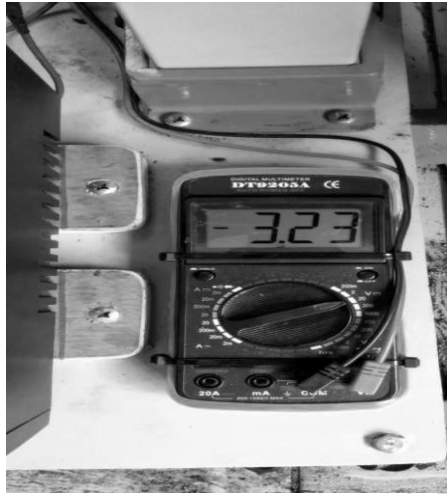
Figure 25: Multimeter voltage output with load (battery)
