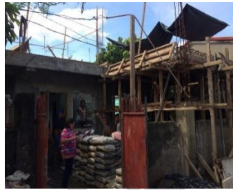
House built on mixed concrete
