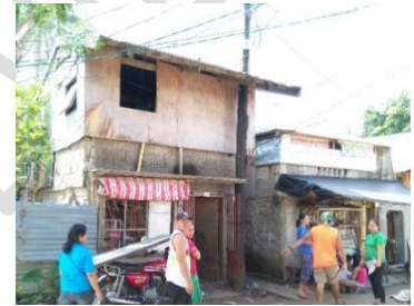
Poor building design
