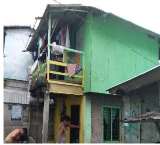
2. Mixed Concrete & Lumber
