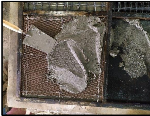
c. shows casting of the top skin ferrocement layer.
