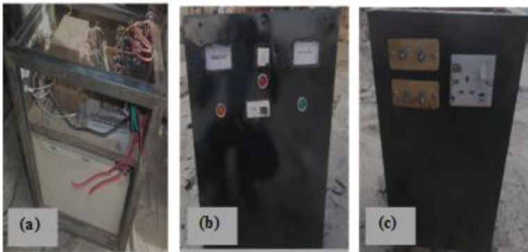
Fig. 3. The Inverter used: (a) Batteries connection, (b) Front view and (c) Rear view
