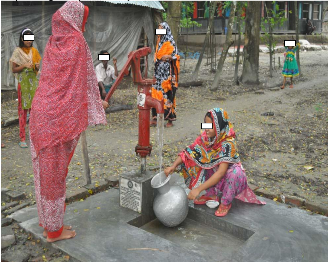
Figure 4: Tube well with on high ground with cementing base [24]
