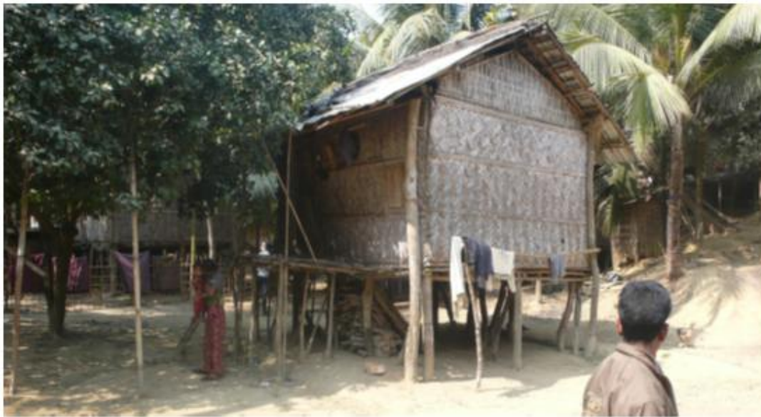
Figure 1: Flood resistant housing in Bangladesh [16]
