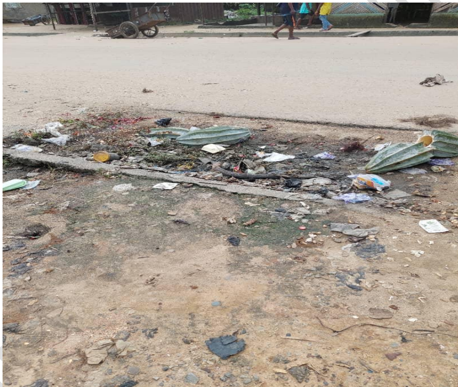
Plate 1: Debris filled drainage in Umuechem Community causing flooding on the adjoining Farmlands Source: Authors' Fieldwork, 2022
