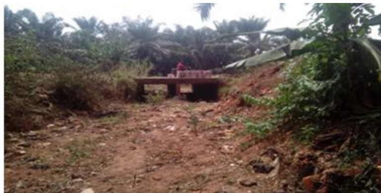
Plate F: The same gully erosion at Onuiyi Road Culvert in 2020 (Note the house around the gully site, with the height of the house about half of the gully depth at 3.84 m)
