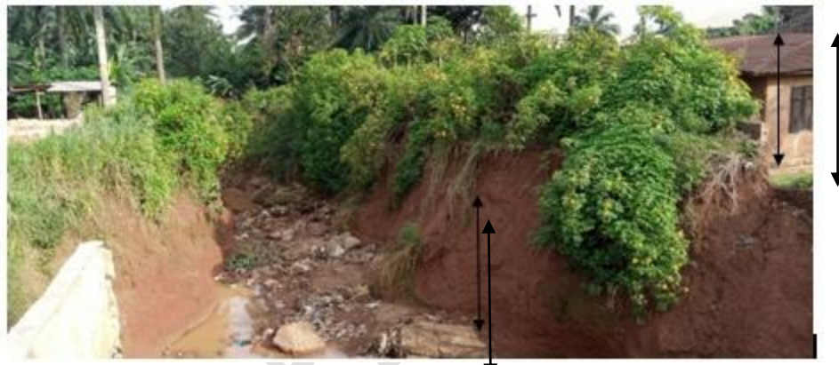
Plate F: The same gully erosion at Onuiyi Road Culvert in 2020 (Note the house around the gully site, with the height of the house about half of the gully depth at 3.84 m)
