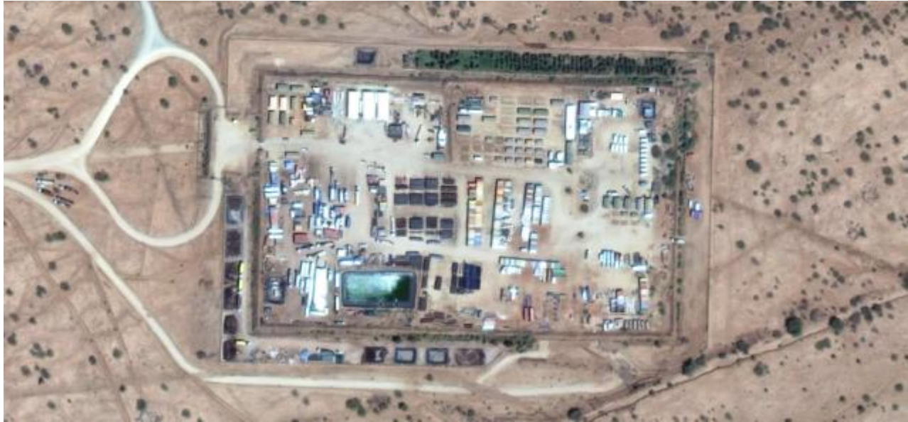
Figure 2: Satellite picture of rig site (Source; Google maps)
