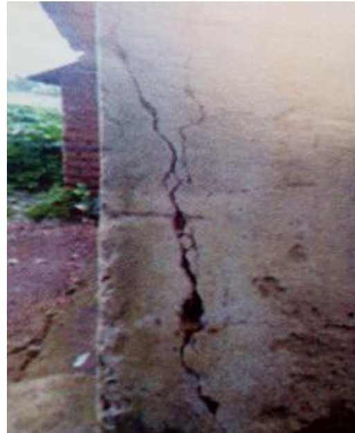
Figure 1: (a) Field photograph of cracked wall observed at Mpape area (b) Field photograph of cracked wall observed at Kwoi area
