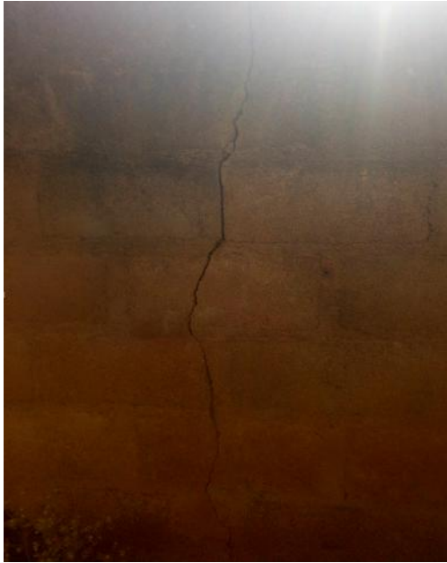
Figure 1: (a) Field photograph of cracked wall observed at Mpape area (b) Field photograph of cracked wall observed at Kwoi area
