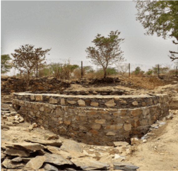
Plate 7: Open well situated at farm of Farmer C
