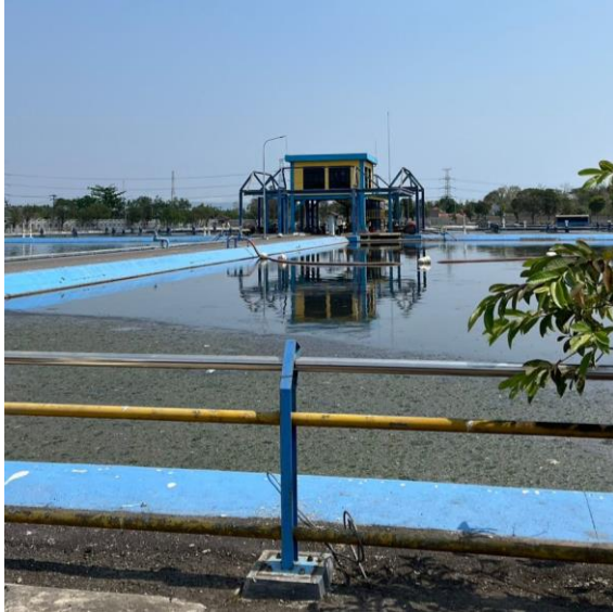
Figure 1. Sewon WWTP in October 2023
