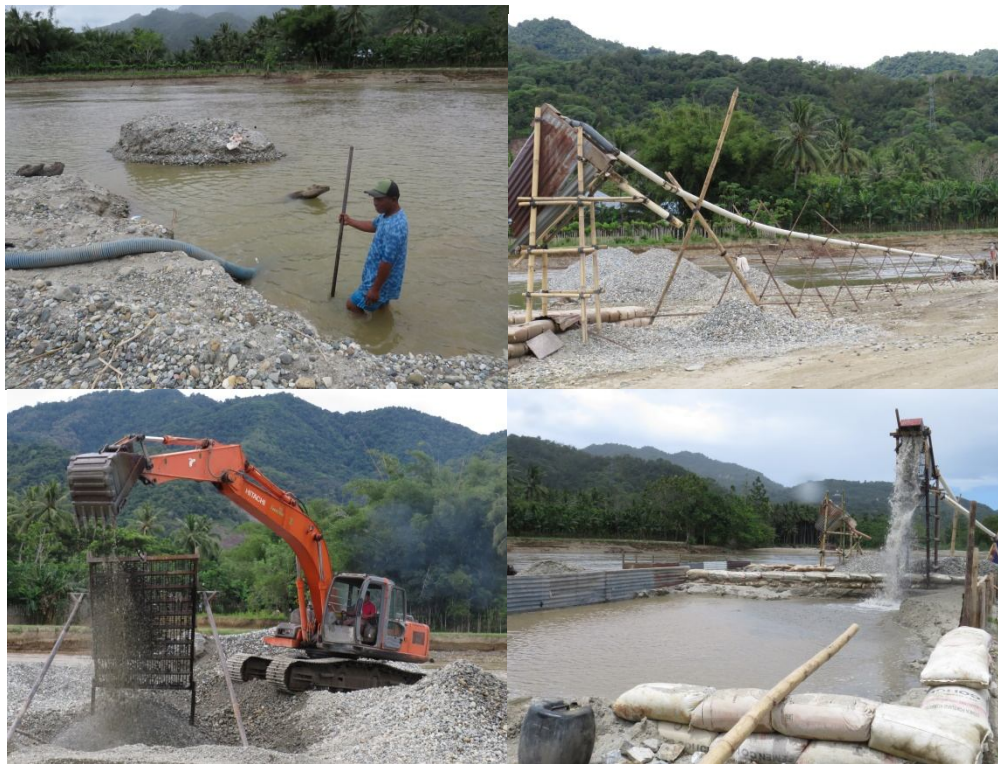
Figure 2: Sand excavation process
