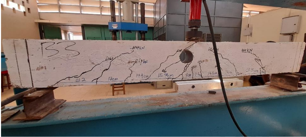
Fig. 6: 3-point loading test of RC beams with openings embedded with PVC pipes
