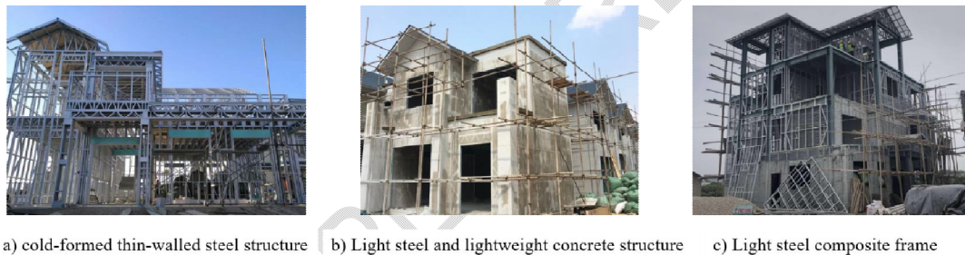
Figure 1 Prefabricated light steel composite structure system (a,b&c )
