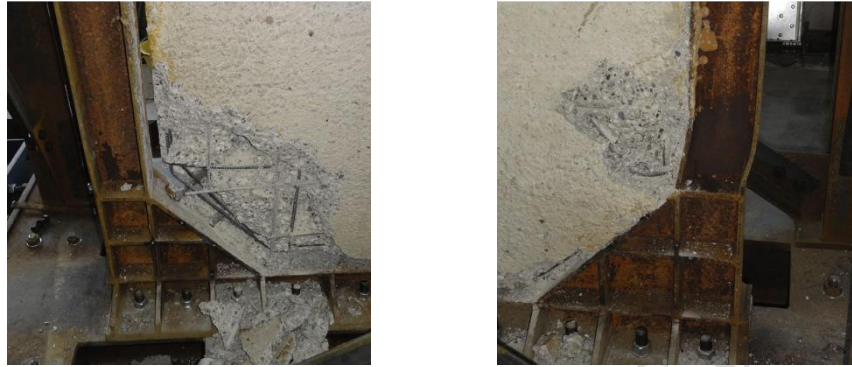
Fig3 Failure mode of SRCW specimen
