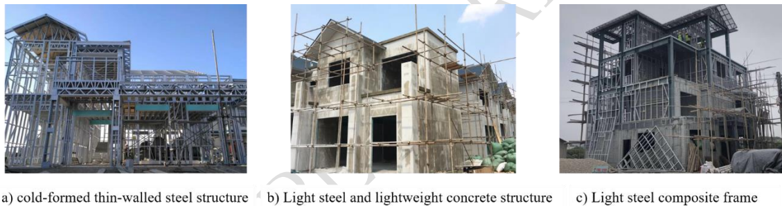
Figure 1 Prefabricated light steel composite structure system
