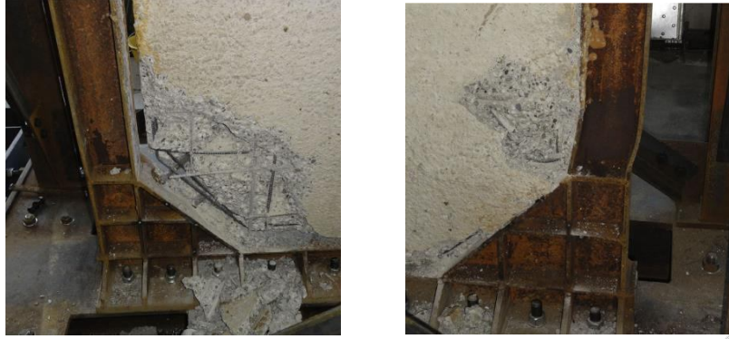
Fig. 5 Failure mode of SRCW specimen
