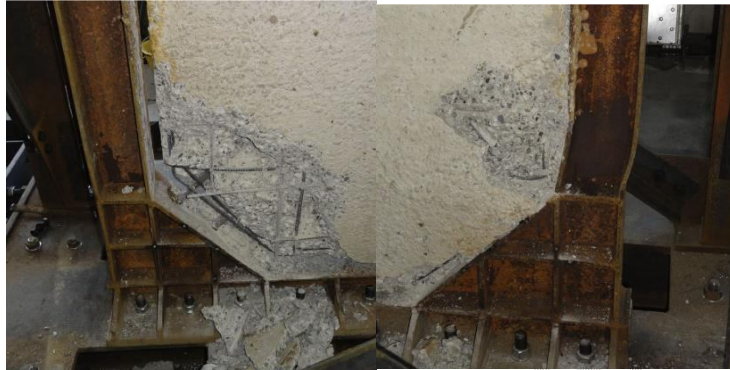
Fig. 5 Failure mode of SRCW specimen
