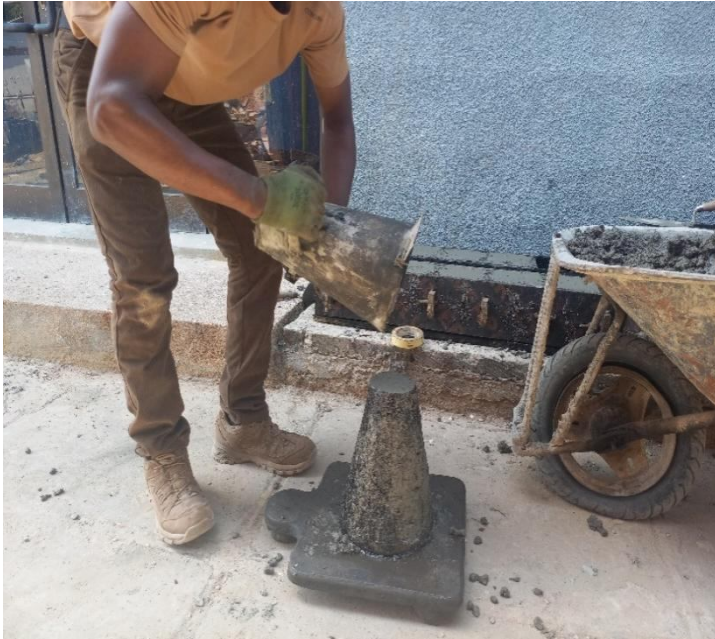
(a) Slump Test on the Fresh Concrete.
