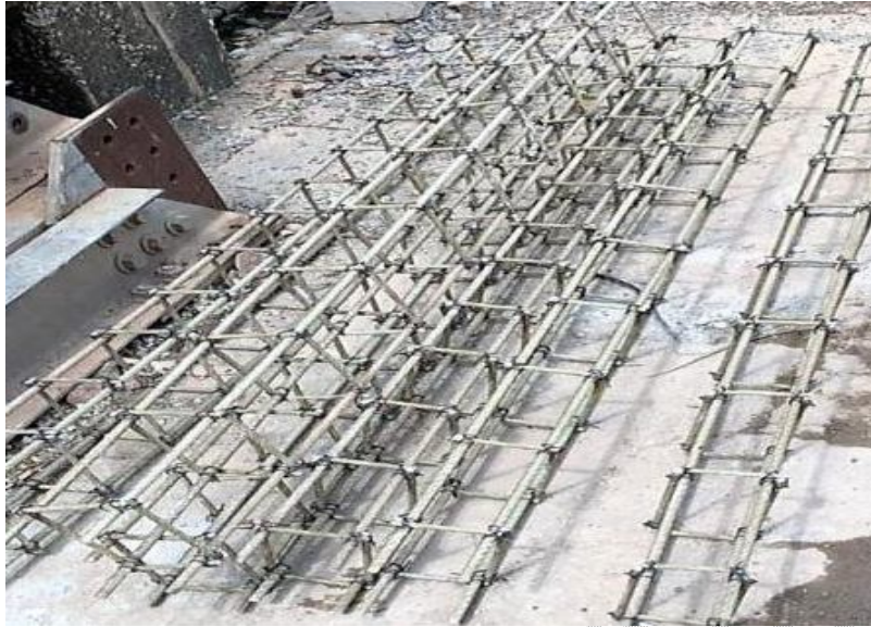
(c) Fabricated GFRP cages
