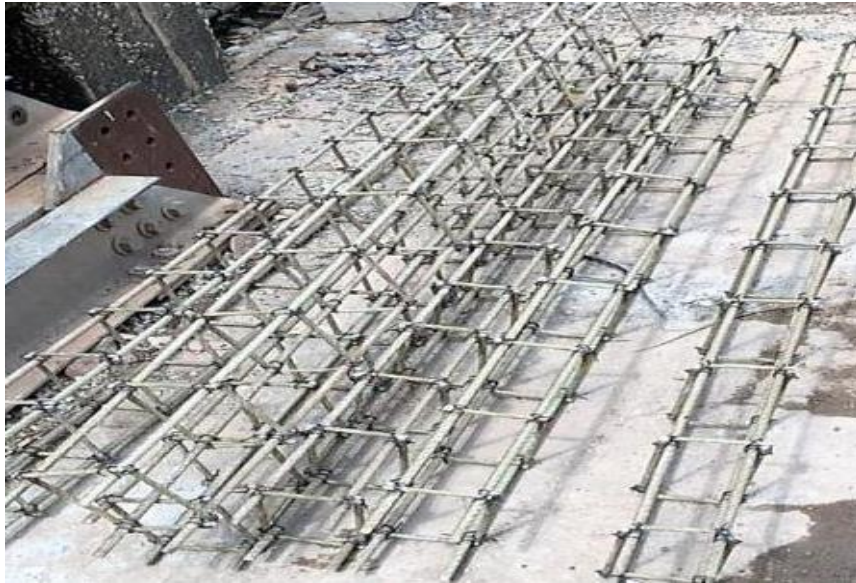
(c) Fabricated GFRP cages
