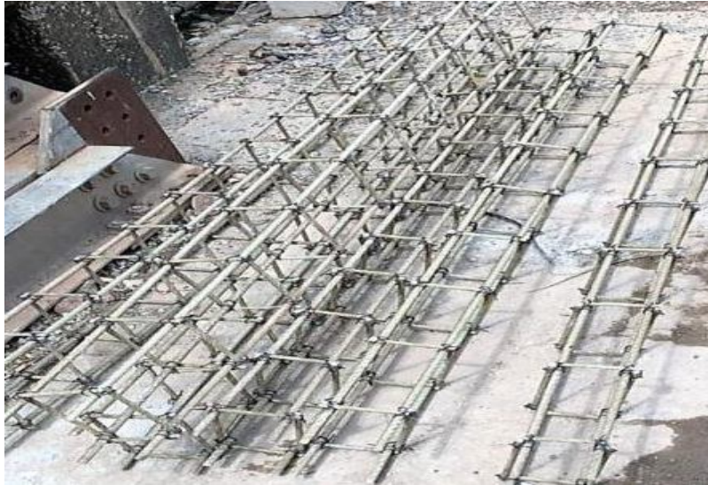
(c) Fabricated GFRP cages
