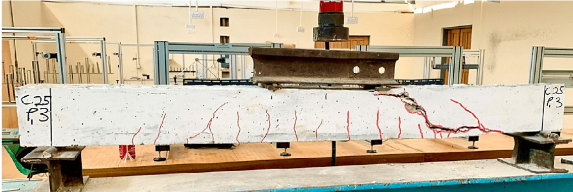
Fig. 11. Beam C25/ \rho_3 failure mode
