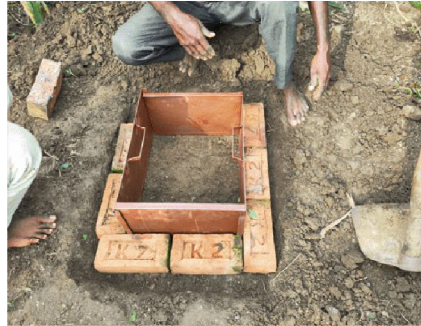
5. Iron plank and Frame Placement
