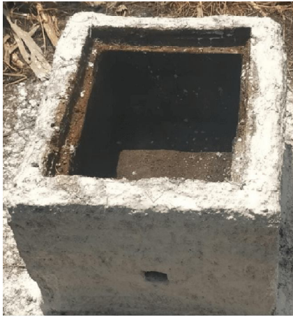
11.Repairs and Cleaning
