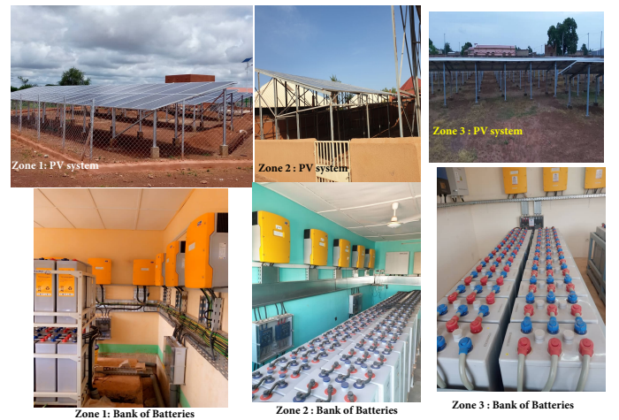
Figure 6: 50kW_p power plant installed in the three climatic zones of Burkina Faso
