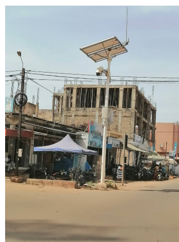
Figure 1: Surveillance camera powered by PV energy to control road traffic in the City of Ouagadougou (Burkina Faso)
