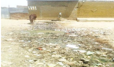
Figure 4 : Drilling with the presence of livestock and wastewater
