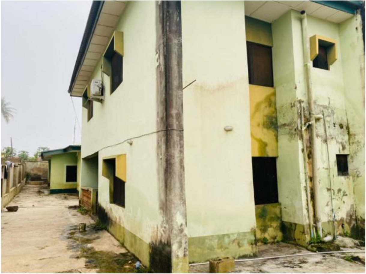
Plate 7: Plumbing defect
