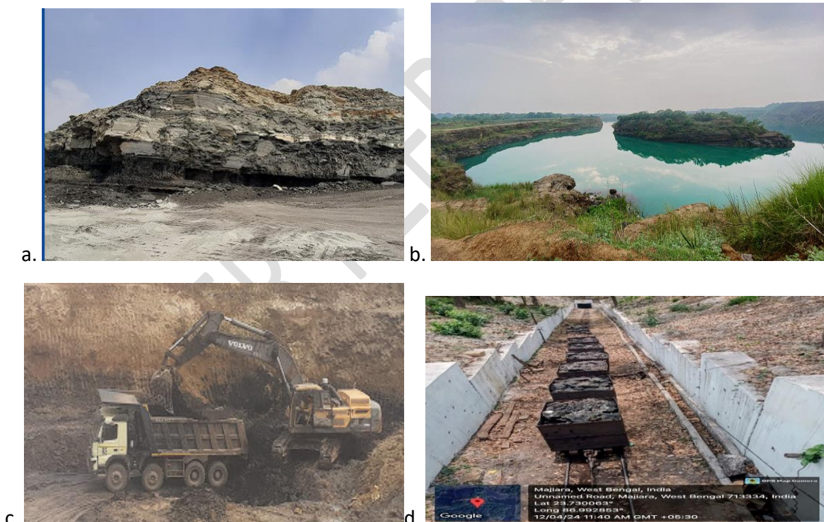
Fig 5(a): The project area Bhanora OC patch (b) The drainage system (c)The coal mines / the OB area (d) Waterlogged area in Sripur e. Loading source of air pollution (f) Transportation
