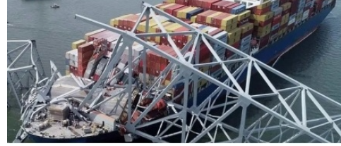
(b) The collapsed Baltimore bridge in USA
