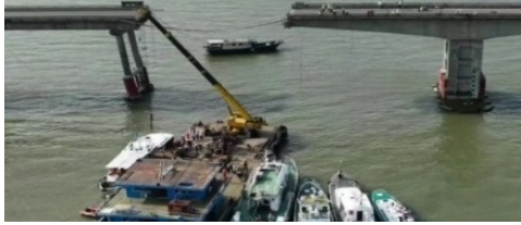
(a) The collapsed Lixinsha bridge in China
